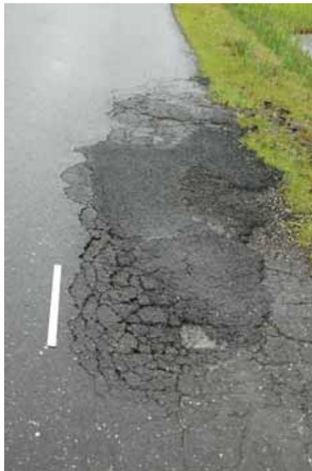
*Typical Paved Road Deterioration*
